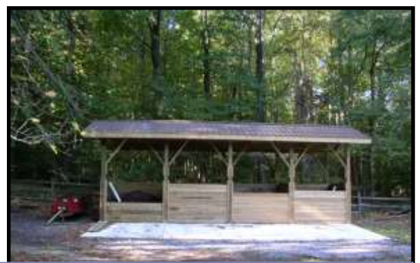
Covered Manure Storage Facility
